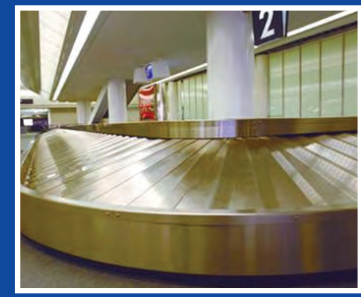
Airport Baggage Handling
